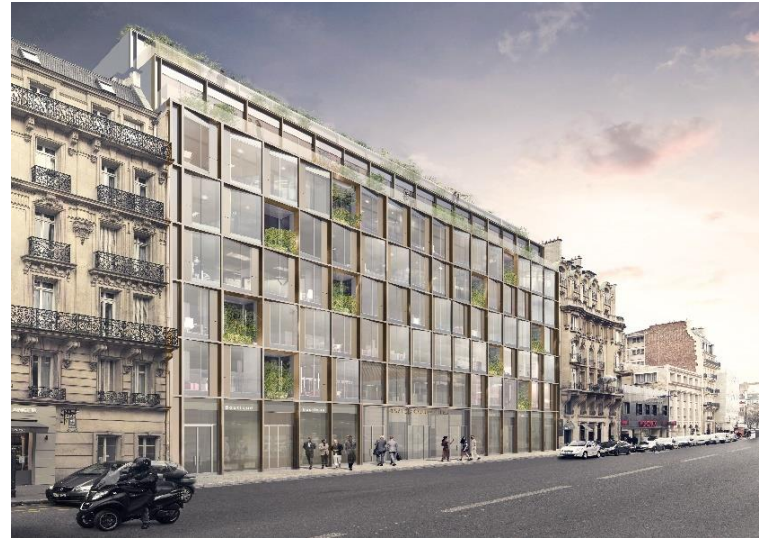
80 METERS OF FACADES ALONG COURCELLES STREET
